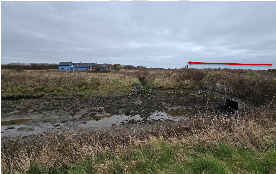
Figure 4-20 Alignment of Greenway traveling over the existing bridge on the L6090 Carrowncalla
