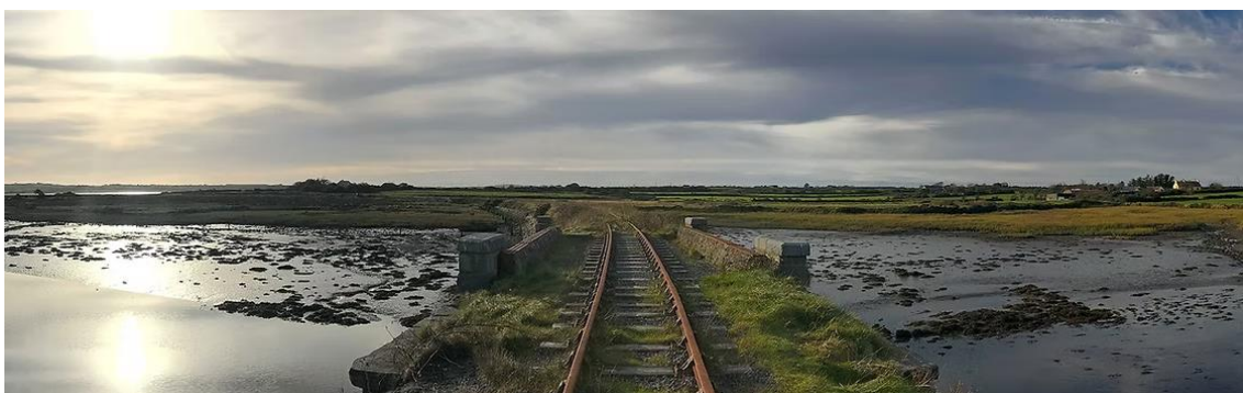
Figure 4-14 Existing Railway Bridge at Moyasta looking west
