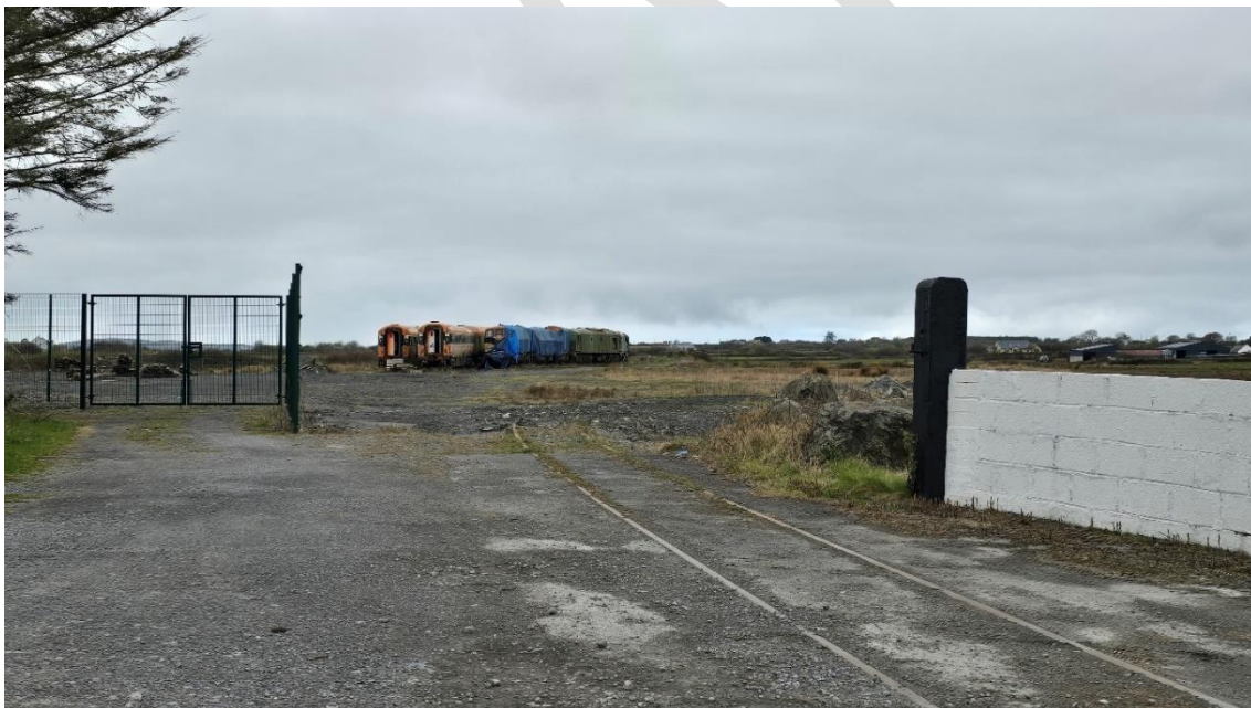
Figure 4-16 Existing tracks along the former railway line along which the proposed greenway will run on the approach to Moyasta village
