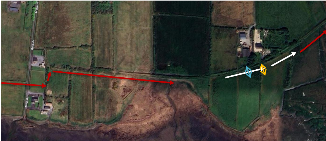
Figure 4-12 Location of retaining wall marked in white arrows, overpass in blue and footbridge in orange
