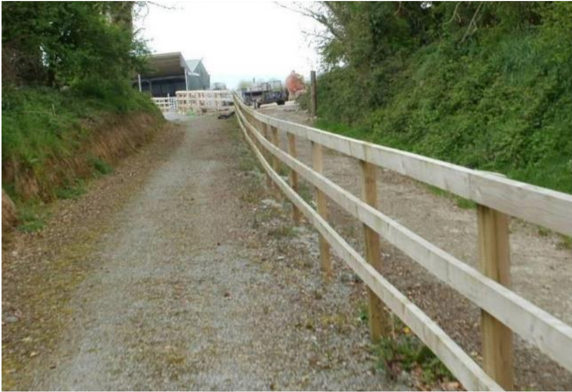
Figure 4-38 Greenway with a parallel farm access track (GST Limerick)
