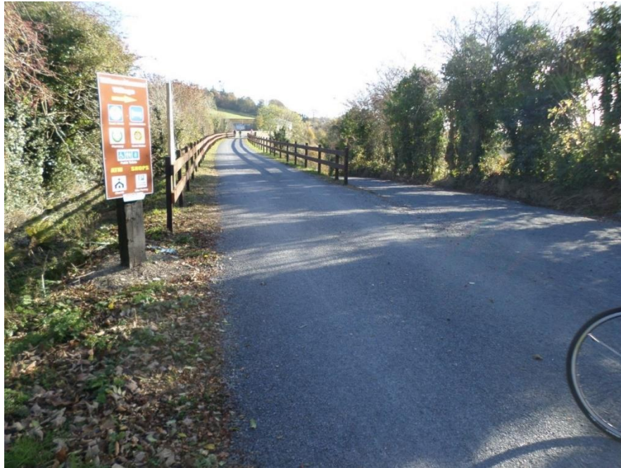
Figure 4-43 Example of boundaries. (Location: the Waterford Greenway)
