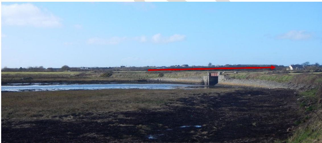
Figure 4-13 View north towards existing Railway Bridge ("Red Bridge") at Moyasta
